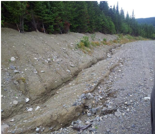
Figure 1: Sheet, rill and gully soil erosion that could have been prevented with adequate cross drainage, vegetation and a soil scientist's understanding of soil and water.
